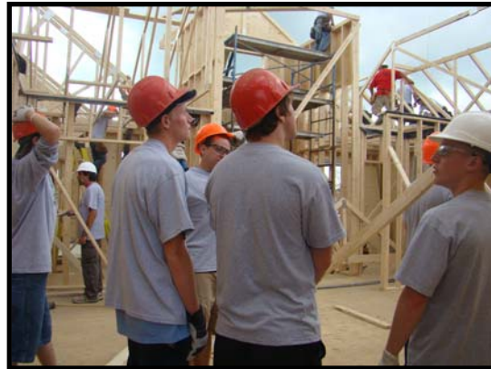
KDHS Students were at the centre of Kingsville's Extreme Build project
