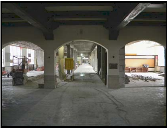
View from main lobby down west corridor
